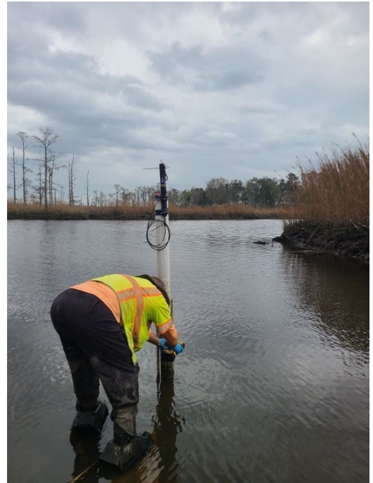
Equipment installation in the marsh
