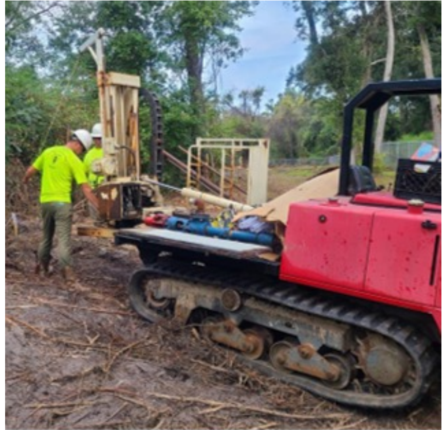
Monitoring Well Installation
