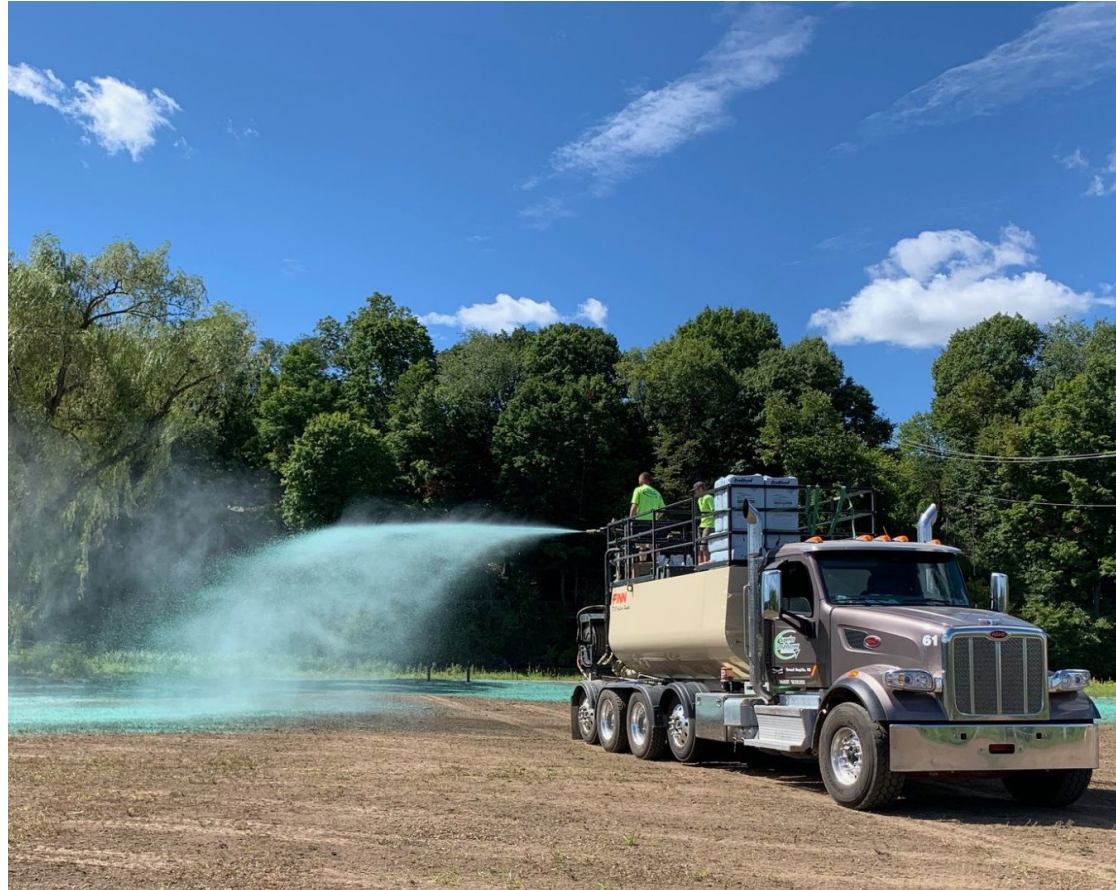
Example of hydroseeding to restore vegetation
